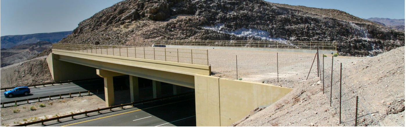
This is one wildlife overpass on US 93, about 3 miles from the Hoover Dam. This overpass provides safe passage to desert bighorn sheep and other wildlife
